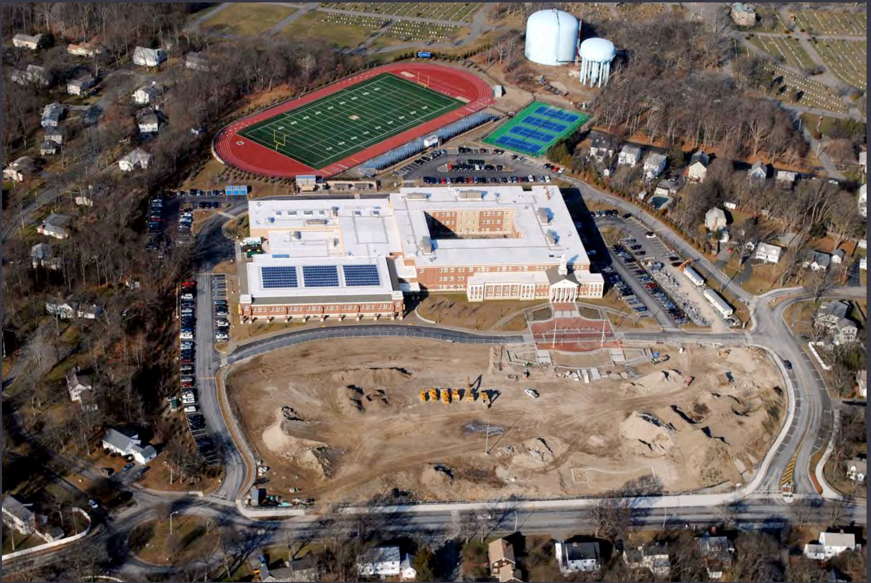
Norwood High School - After to demolition of old H.S.
